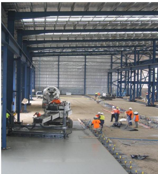
Shepherd Contracting are the concrete placers and are using the Somero Laser Screed to place and finish the slabs. Because Fibercon was specified it means that the contractor can place the slab straight from the truck, eliminating a concrete pump. This is a massive saving on such a large project.
