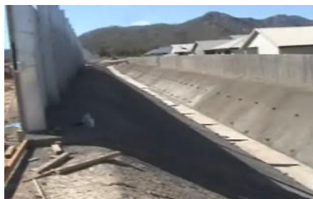
V-Drains, Large Drains, Channels
