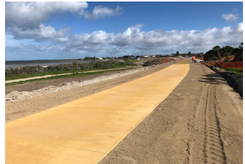
Photos of the Shared Pathway under construction, and the completed outcome
